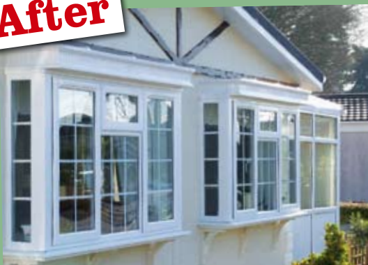
A close-up of the new uPVC-framed windows which are fitted with Georgian glazing bars
