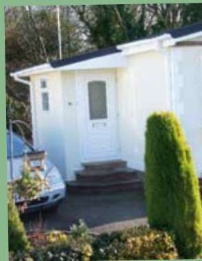
The porch exterior now matches the rest of the home
